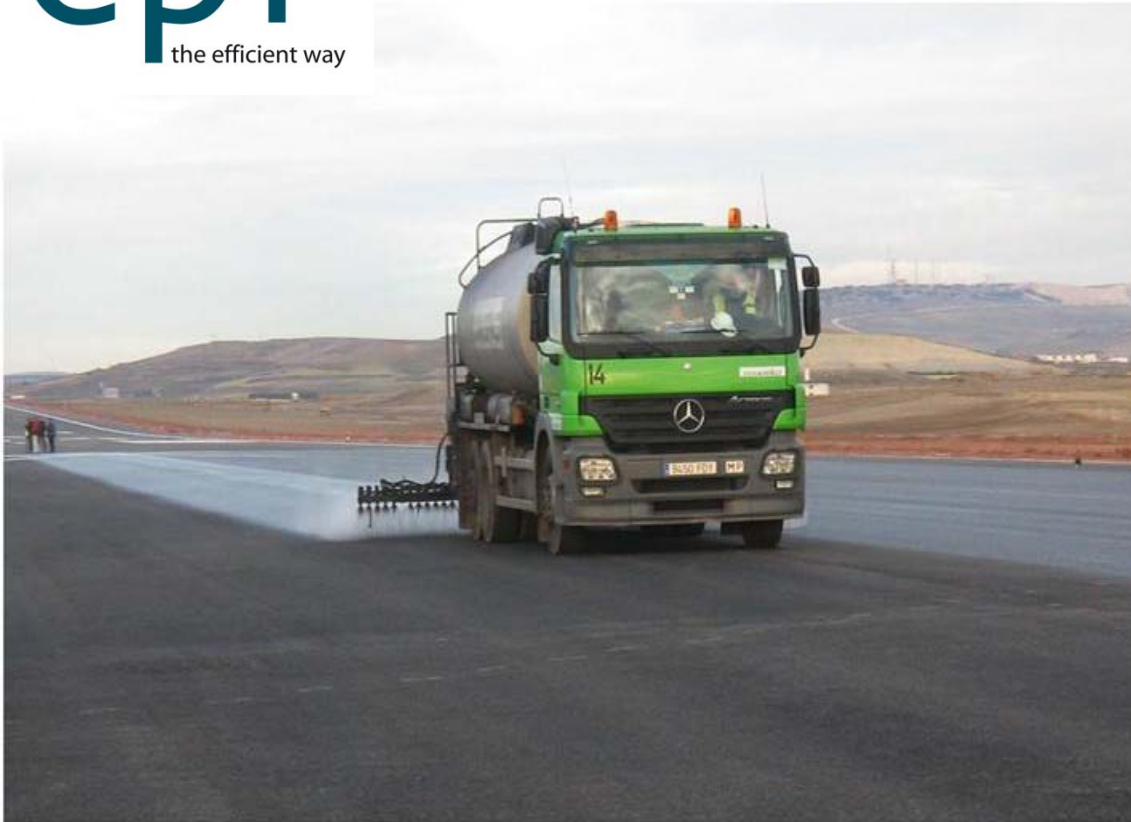
Distributor applying tack coat
